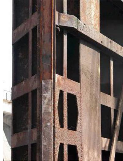
FIGURE 3: Quoin block failure.
