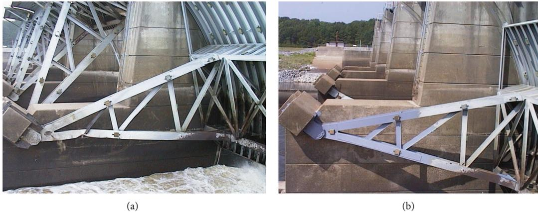
FIGURE 5: Tainter gate with strut arm damage from barge impact before and after repairs.
