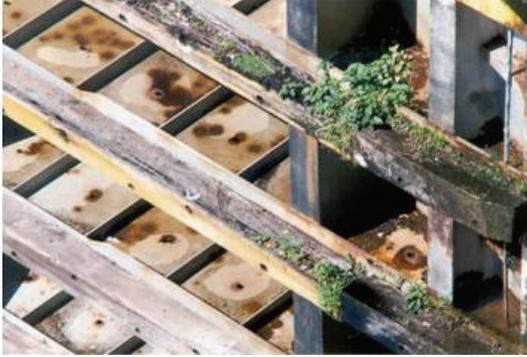
FIGURE 1: Corrosion on a miter gate.
