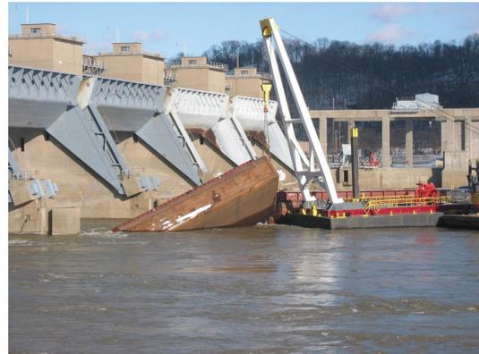
FIGURE 4: Barge impact at Belleville Locks and Dam.
