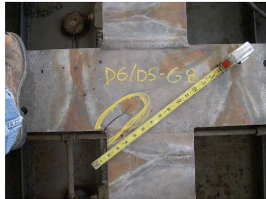
FIGURE 7: Fatigue crack in girder flanges of miter gate.
