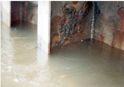
FIGURE 2: Corrosion inside a lock miter gate compartment.
